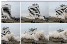
Collapse due to wind load
